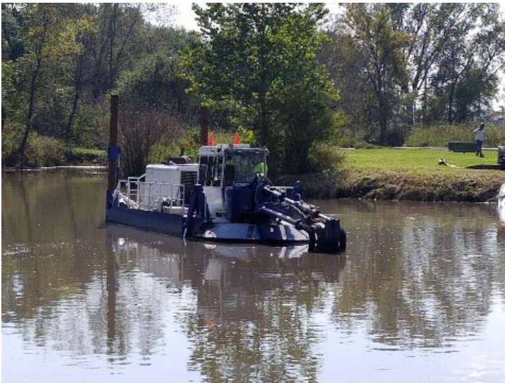
Hydraulic dredge removing legacy sediments from Token Creek.
